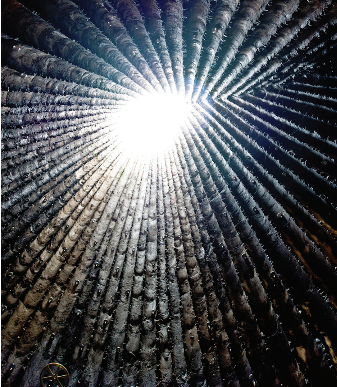
Figure 69: Interior of the Bruder Klaus Chapel (2007) by Peter Zumthor showing the hollow blackened cavity and charred walls.
