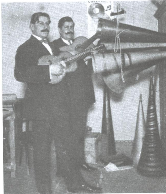
This photo, taken in a recording studio circa 1915, shows two "payadores" recording in front of large horns that conducted the soundwaves through a wall to the technician on the other side. All of the recordings done by Barrios during the period 1913-1924 were done thusly with acoustic technology.
