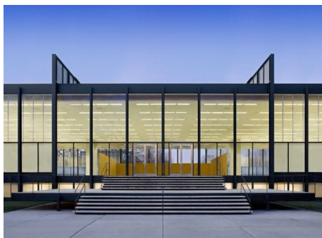
Crown Hall, Chicago, USA 1956
